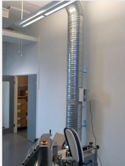
Picture 2 .The air suction line equipped with Genano technology® and filter
